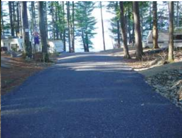
Same road, resurfaced, crowned and ditching/turnouts added #2, 12, 15, 16
