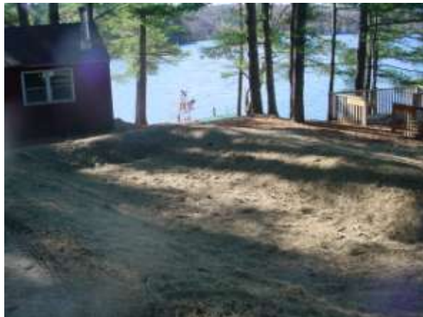
Underdrain filter swale & site of future shrub plantings
