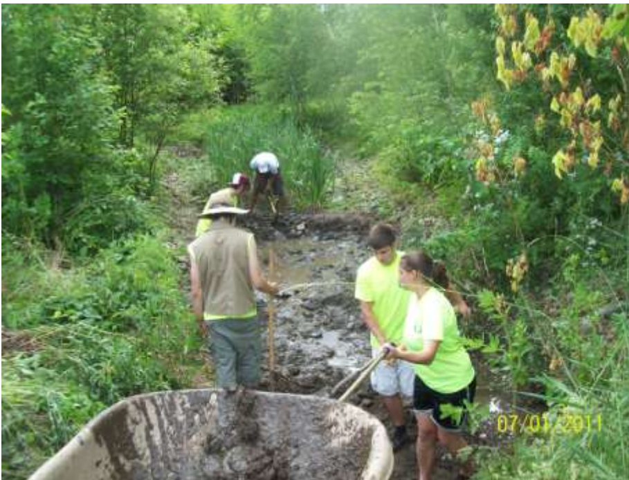
Figure 2 - Route 32 Plunge Pool - After (hauled away 4 yards of sediment)
